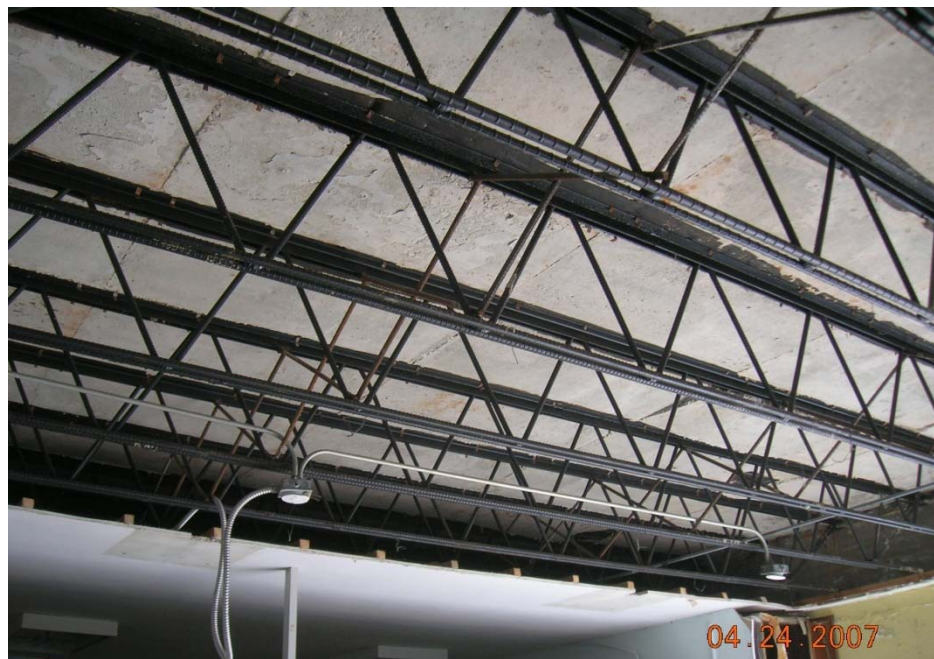
Figure 36 – Test Site: Open-Web Joists
