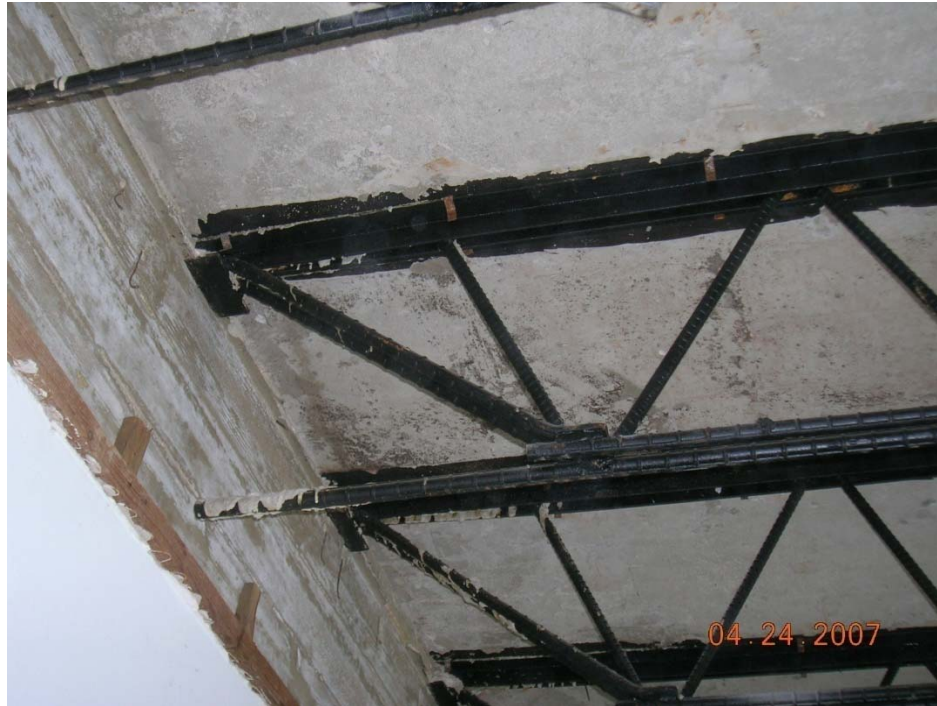
Figure 37 – Test Site: Open-Web Joist Support
