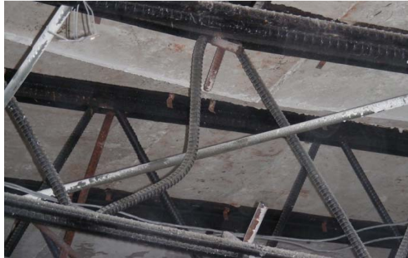
Figure 89 – Buckling Failure
