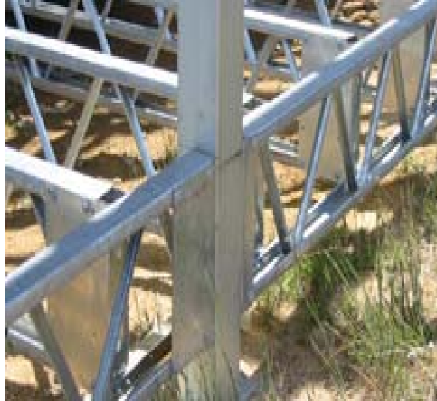
Figure 15 – Hopleys Domestic Flooring (Hopleys, 2006)
