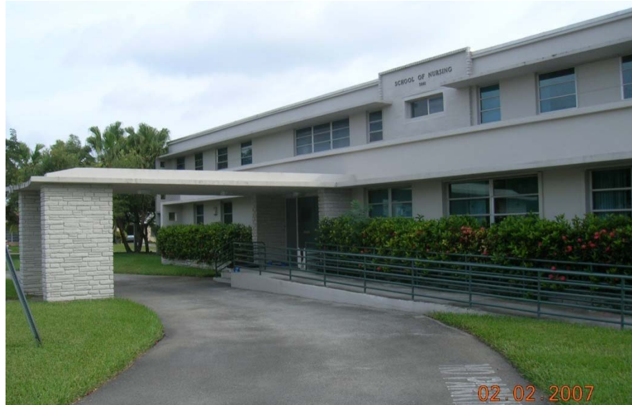
Figure 35 – Test Site: School of Nursing Building
