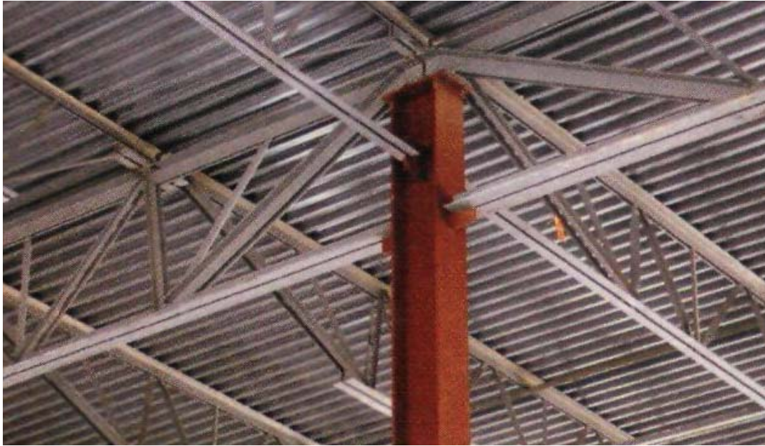
Figure 5 – Steel Joist – Column Connection (Hopleys, 2006)
