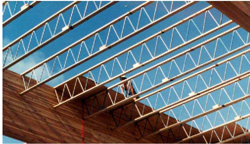
Figure 4 - Light-Weight Floor System (Hopleys, 2006)
